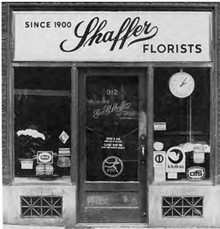
The original form and features of this 1920s storefront have been retained through Preservation. Photo: David W. Look, AIA.
