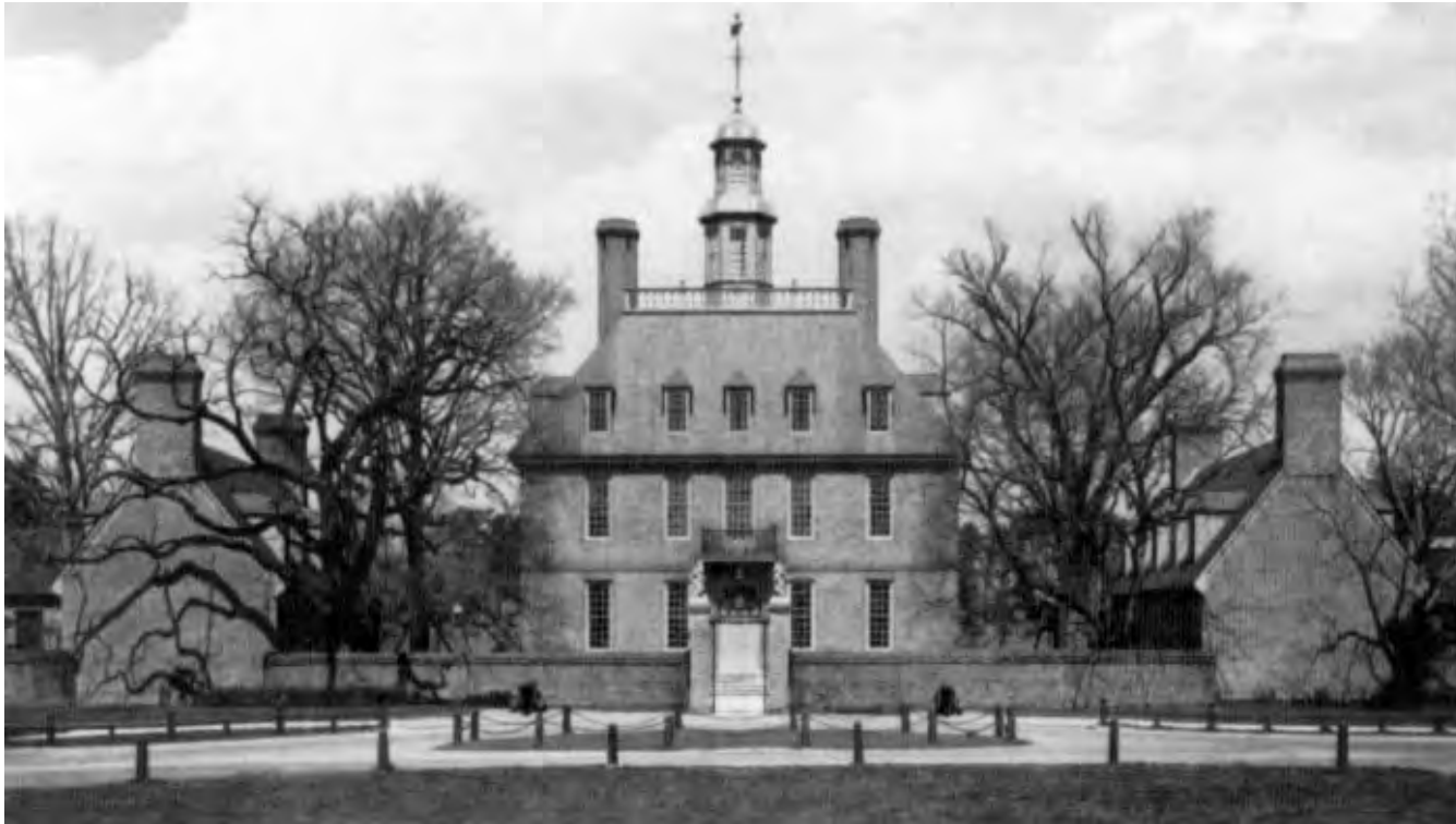
In the 1930s reconstruction of the 18th century Governor's Palace at Colonial Williamsburg, Virginia, the archeological remains of the brick foundation were carefully preserved in situ, and serve as a base for the reconstructed walls. Photo: The Colonial Williamsburg Foundation.
