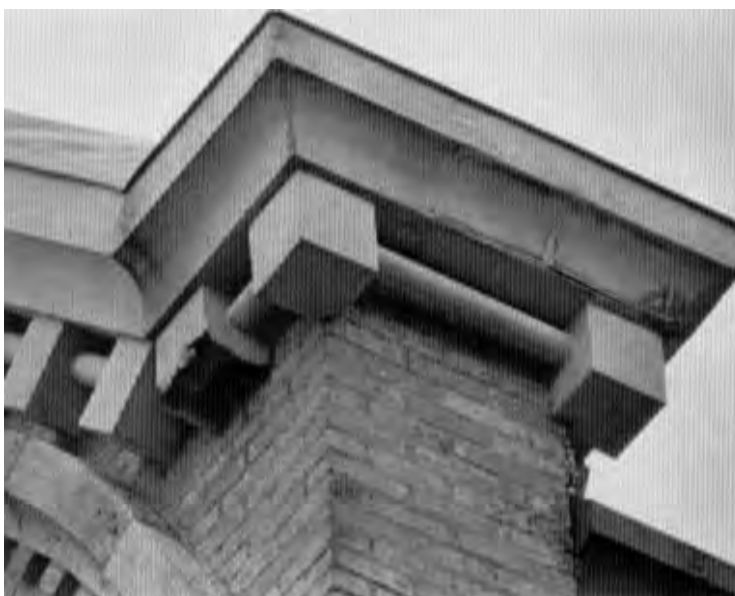
Two examples of “limited replacement in kind” point out an appropriate scope of work within the treatment, Preservation. (a) One metal modillion that has sustained damage from a faulty gutter will need to be replaced; and (b) targeted repairs to deteriorated wood cornice elements (fascia board and modillions) meant that most of the historic materials were retained in the work.
